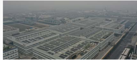
The Distributed Photovoltaic Project in Quzhou Park
