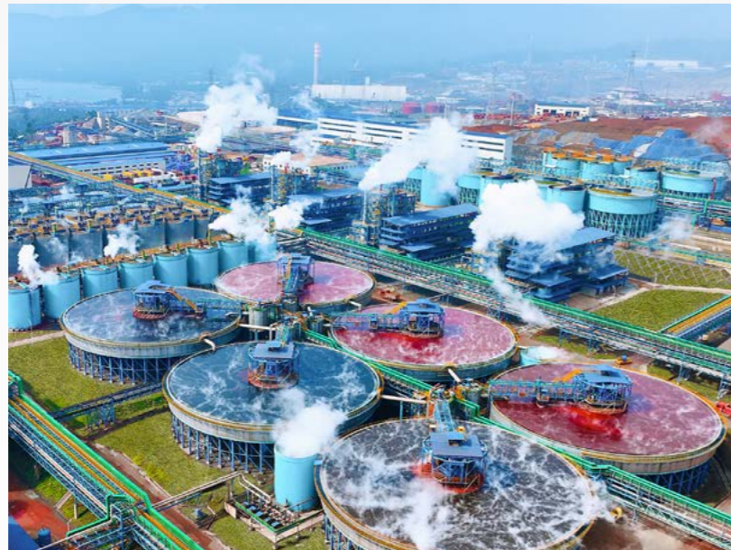
Huayue Project in Indonesia
